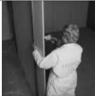
Fasten vertical strut from back side.
