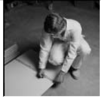
21. Measurements for box opening are then transferred to face of panel.
