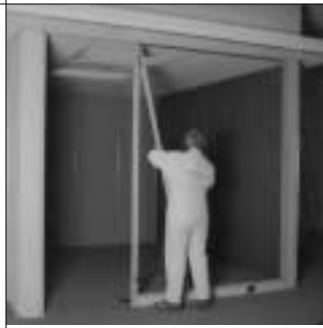
17. After continuous sill rail is installed, AGL-342 door frame glazing cover is secured to door jamb as previously described.
