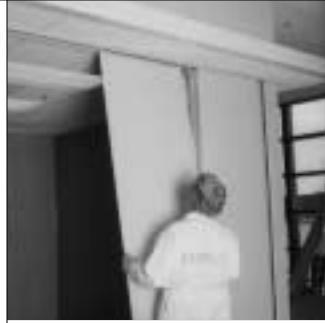
7. Continue installing ULTRAWALL panels and studs...
