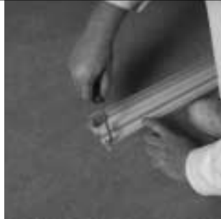
19. SCL-381 mullion clips are screw-attached to both ends of AGL-340 glazing rail.
