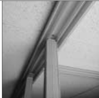
Method 1. Snip aluminum inner flanges to create a notch which will receive strut web.
