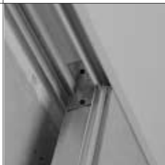
17. Top and bottom of T-studs can be secured with angle clips to increase partition rigidity.
