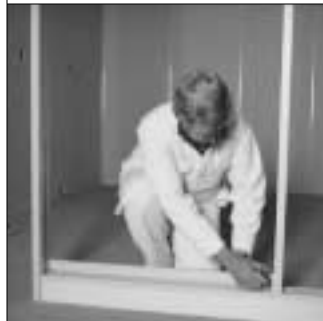
25. Glass stops are marked for tight fit...
