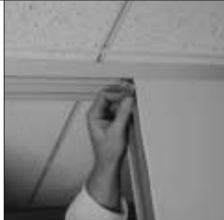
14. Narrow panels adjacent to large openings can be secured with angle clips.
