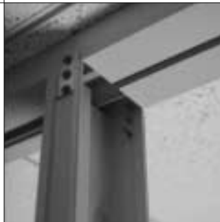
12. Door frame is secured to partition.
