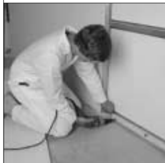
13. 1/4-in. wood strips are applied to face of existing wall to provide backing to panels at base. A 1-3/8"x7/8"x 24 ga. metal is required at the base for fire rated construction.
