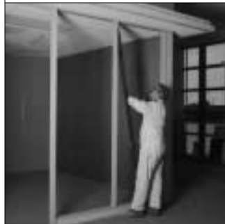
22. AGL-341 glazing cover is snapped into AGL-340 glazing rail to complete mullion.
