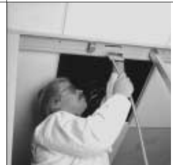
9. Plug-in connector for this type of electrical system is inserted through hole in ceiling runner...
