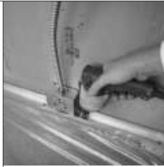
11. Electrical boxes with flanged brackets are easily screw-attached into floor runners.
