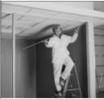
16. Large glass openings divided by vertical mullions require continuous AGL-341 glazing cover to be snapped into ceiling runner.
