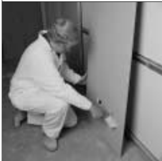
25. Some fabrics may require precutting and removing the fabric to prevent snagging.
