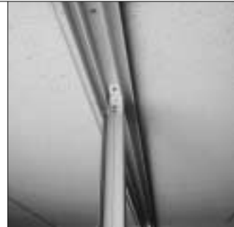
Method 2. Screw-attach sheet metal angle to both ceiling runner and strut.
